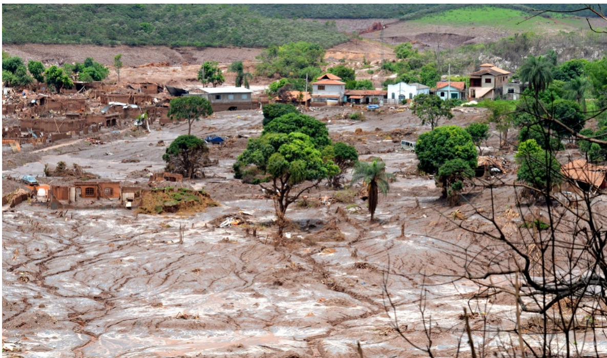
Figure 8. Aftermath of the Fundão tailings dam disaster in Brazil. This mine was a joint venture of BHP. As the dam broke, 45 million cubic meters of iron ore waste and mud covered the nearby town of Bento Rodrigues and beyond. 19 people were killed and at least 60. BHP has previously estimated that tailings would flow about 3.5 kilometers in the event of a potential dam break would flow about 3.5 kilometers. After this very real dam break, the tailings traveled over 600 km, eventually reaching the Atlantic Ocean, illustrating mining company’s history of downplaying risks from their tailings dumps.
